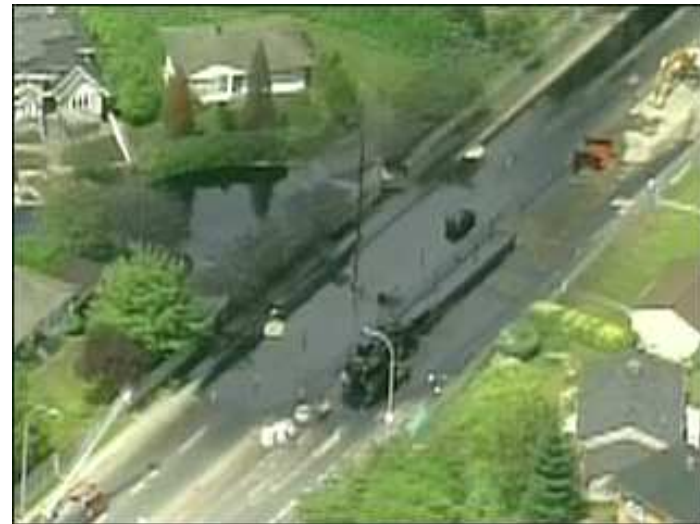
15 th January 2009 Vancouver-line rupture
